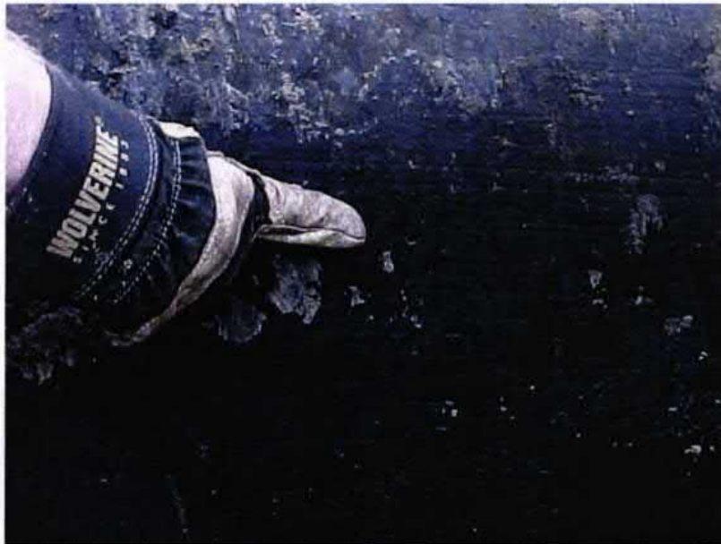
Laural Bay #8 Tank with corrosion and pitting
